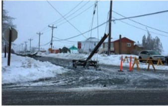
Hydro poles in many areas on the Acadian Peninsula snapped off under the weight of the ice from hours of freezing rain during the storm in late January. (Jane Mather/Radio Canada)
